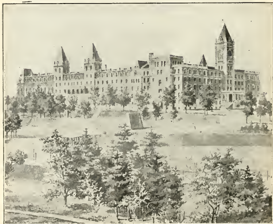
HOLY CROSS COLLEGE, WORCESTER, MASS. A full view from the north.
